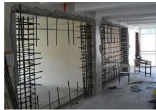
Adding Reinforced Concrete Shear Wall
